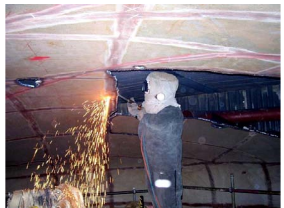
Cutting of Sodium Tanks
